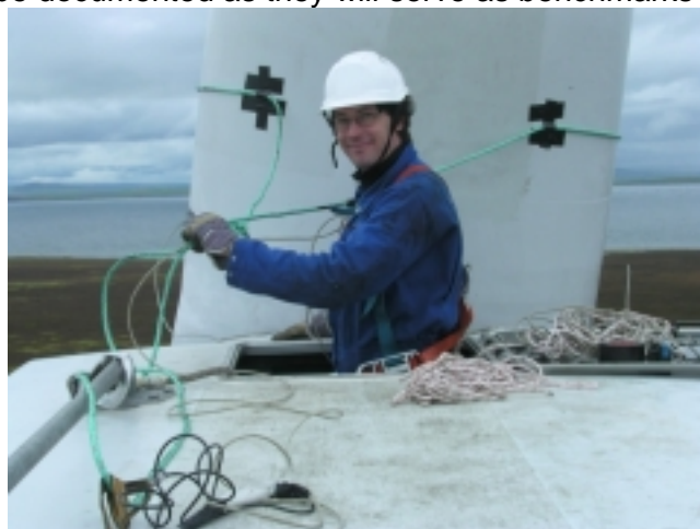
Figure 3 - Dynamic Balancing Set-up
