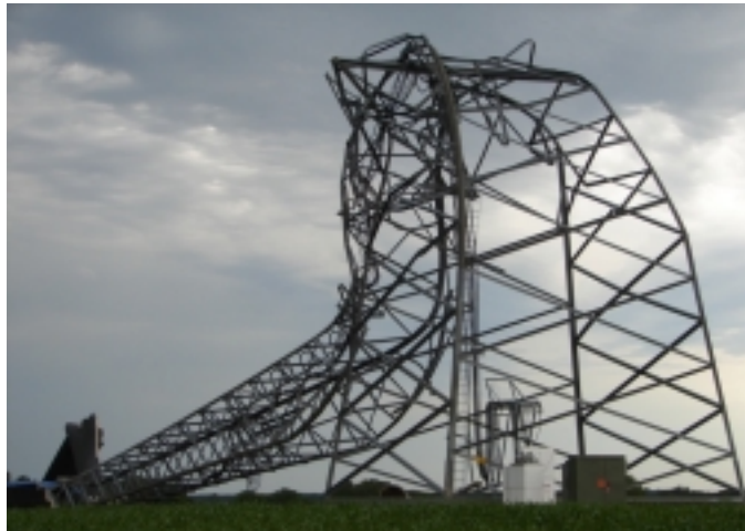
Figure 10 - Catastrophic Turbine Failure
