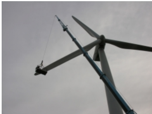
Figure 4 - Man Basket suspended from Crane
